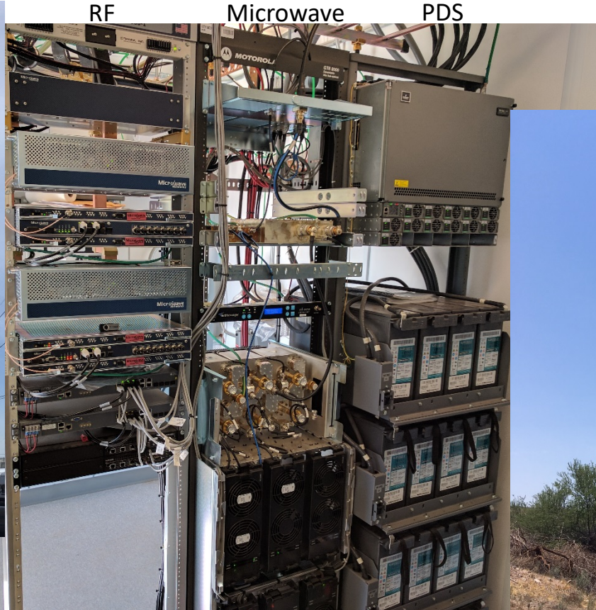
Typical 3-Rack Equipment Configuration
